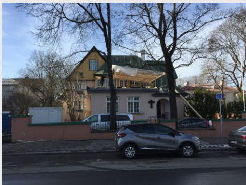
Seminary roof work
